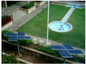
**Caption:** Aerial view of the showcase solar power sub-system designed, built, and installed by SonLight Power at the U.S. Embassy in Tegucigalpa, Honduras. Completed in May 2011, this first-of-its-kind 2-kilowatt grid-tied system will cut the Embassy's carbon emissions by more than 1,000 pounds per year and is a model for visiting dignitaries.
